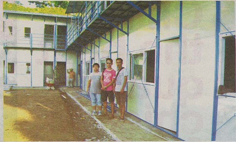
The camp site of the Chinese engineers who are going to work in the Somosomo Hydro in Taveuni. Photo: Seruwaia Waqasaqa
